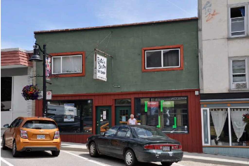
2080 Washington Street in 2019. source: B. Jonker photo
