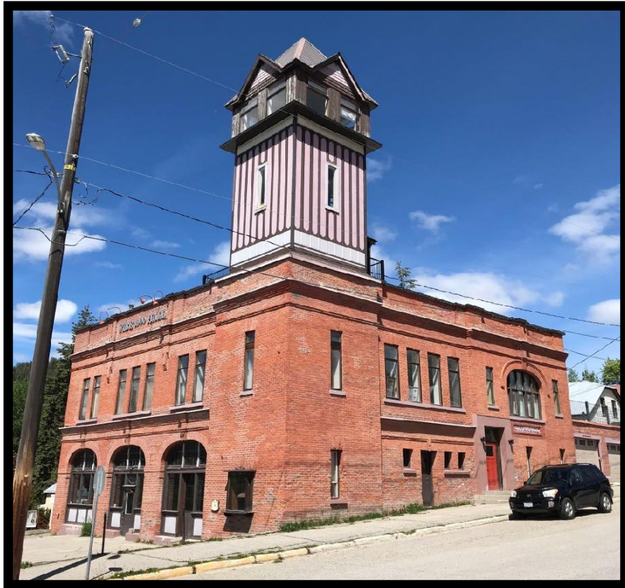
Rossland City Hall/ Fire Hall 2019
