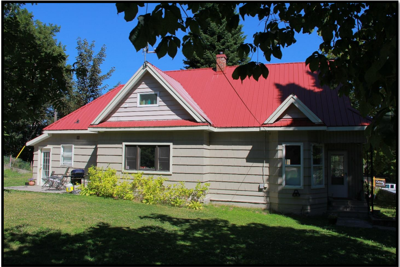
West side of home
