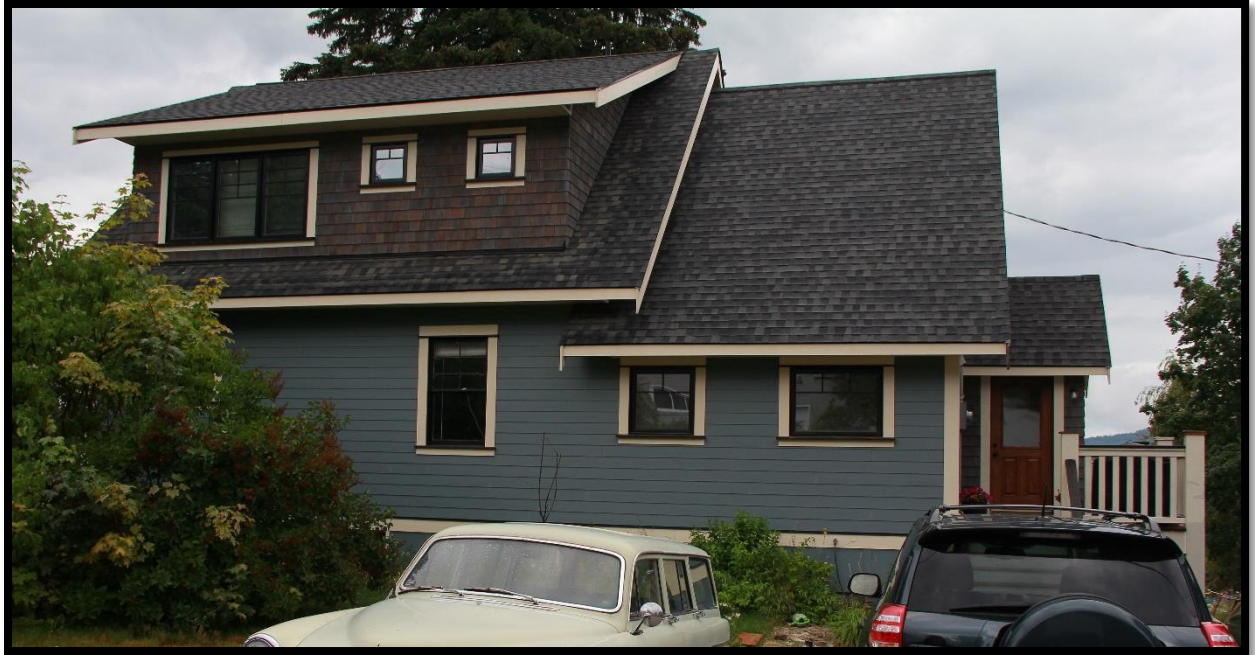
West side of home
