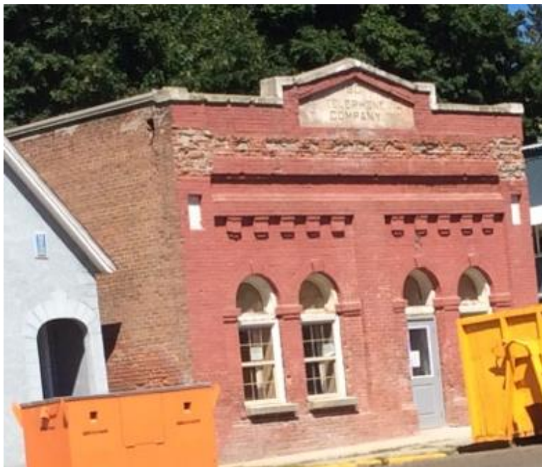
Glazan Block 2017 – restoration in progress
