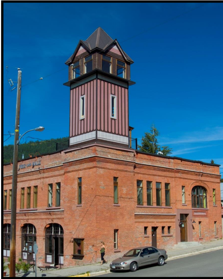
Rossland City Hall/ Fire Hall 2008
