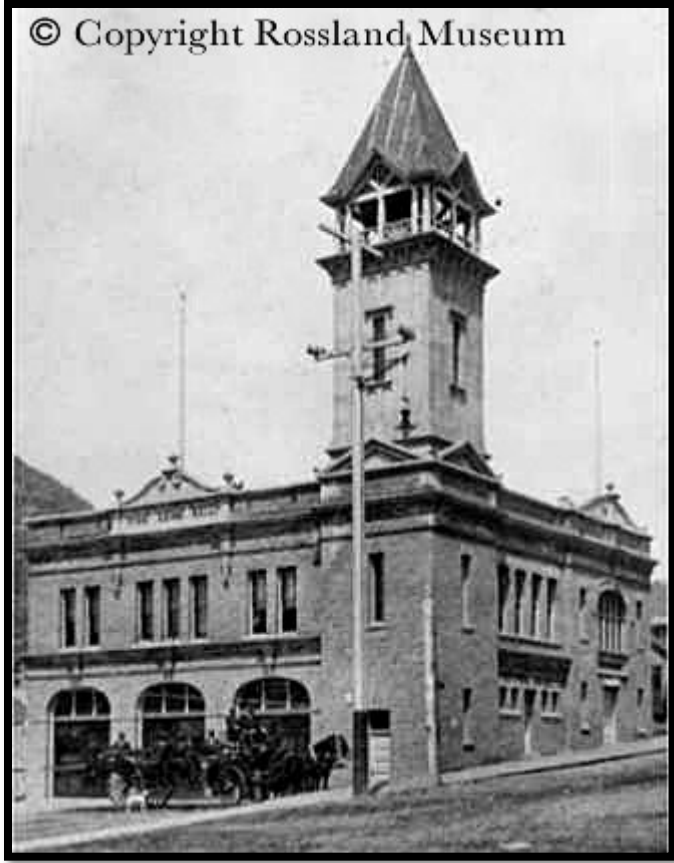
Rossland City Hall/Fire Hall c. 1901
