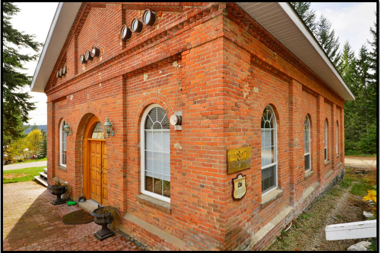
West Kootenay Substation 2014
